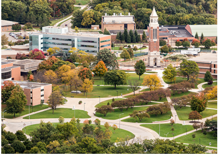
The Oakland Center was closed over the weekend due to a water main break, but is now open and available to the campus community.
